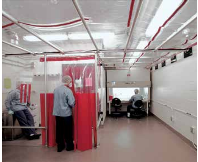
Architecturally Renovated Containment Room
