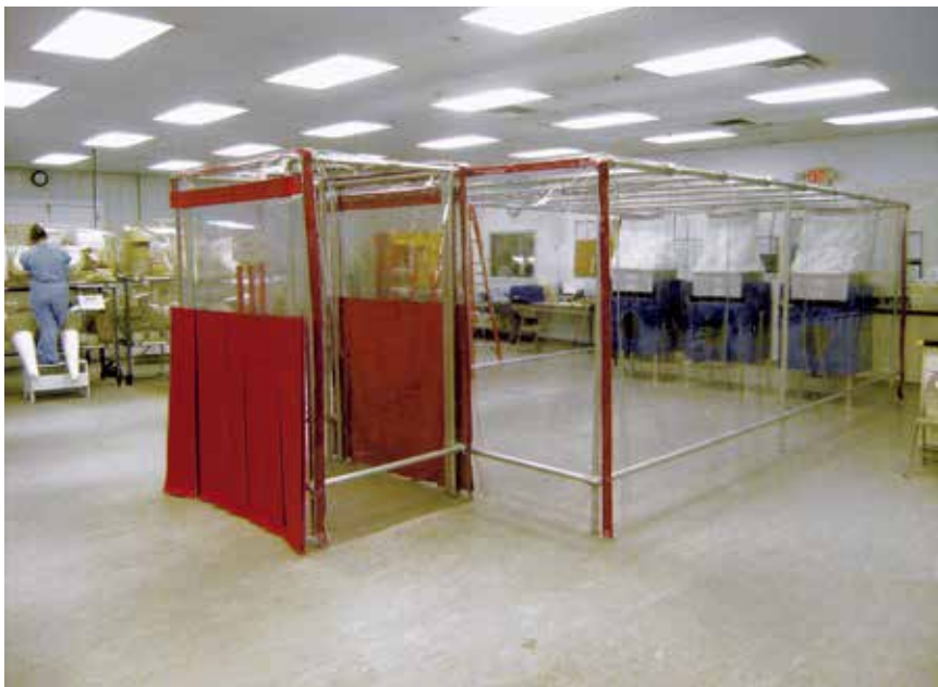
< FREESTANDING NEGATIVE PRESSURE CONTAINMENT ENCLOSURE
