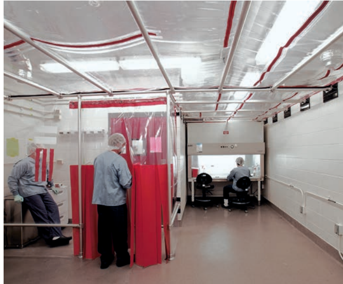
Architecturally Renovated Containment Room
