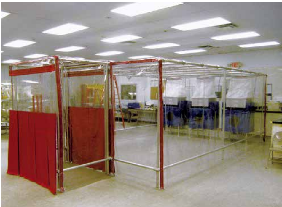
< FREESTANDING NEGATIVE PRESSURE CONTAINMENT ENCLOSURE
