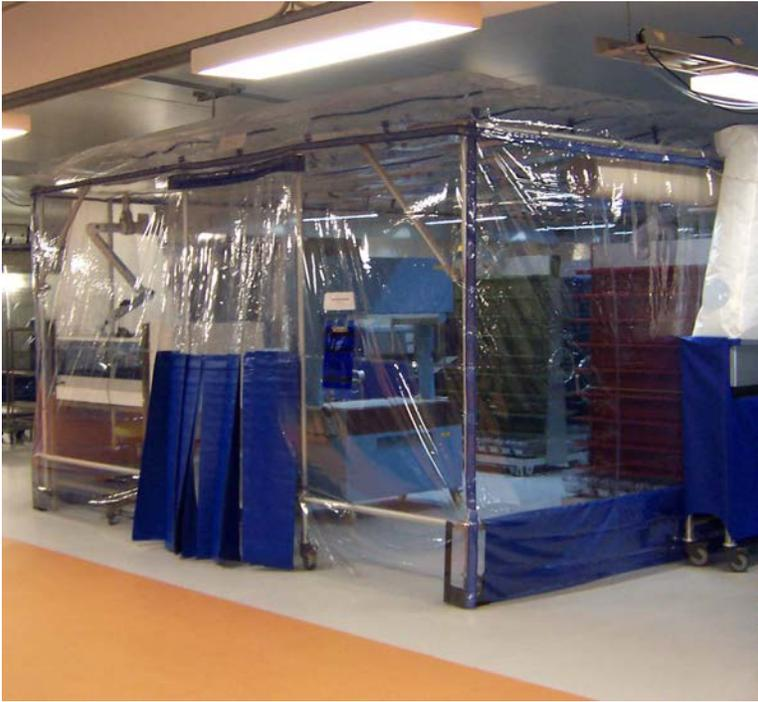
Each bioBUBBLE Enclosure has the capacity to house 1,600 cages in individually ventilated rack systems.
